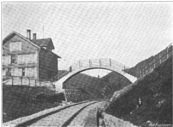
Fig. 34—FOOTBRIDGE AT Km. 3.67
