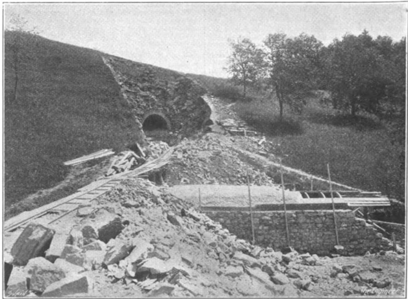
FIG. 52—BRIDGE AT Km. 1.78
