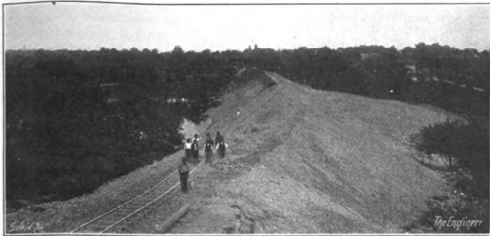
Fig. 7—SLIP ON THE HOHENBÜHL BANK
