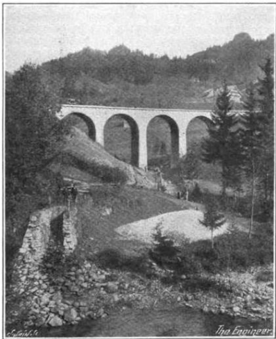
Fig. 4—VIADUCT AT KM. 3.05
