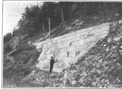
FIG. 26—DRY STONE RETAINING WALL
