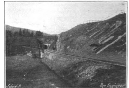
Fig. 13—SLOPE WITH CONCRETE BLOCKS
