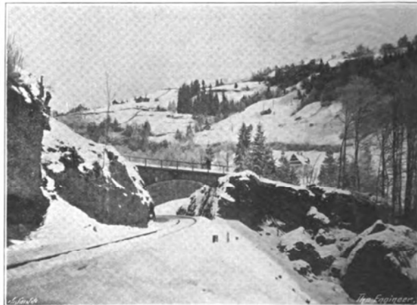
Fig. 35—ROAD BRIDGE AT Km. 5.26
