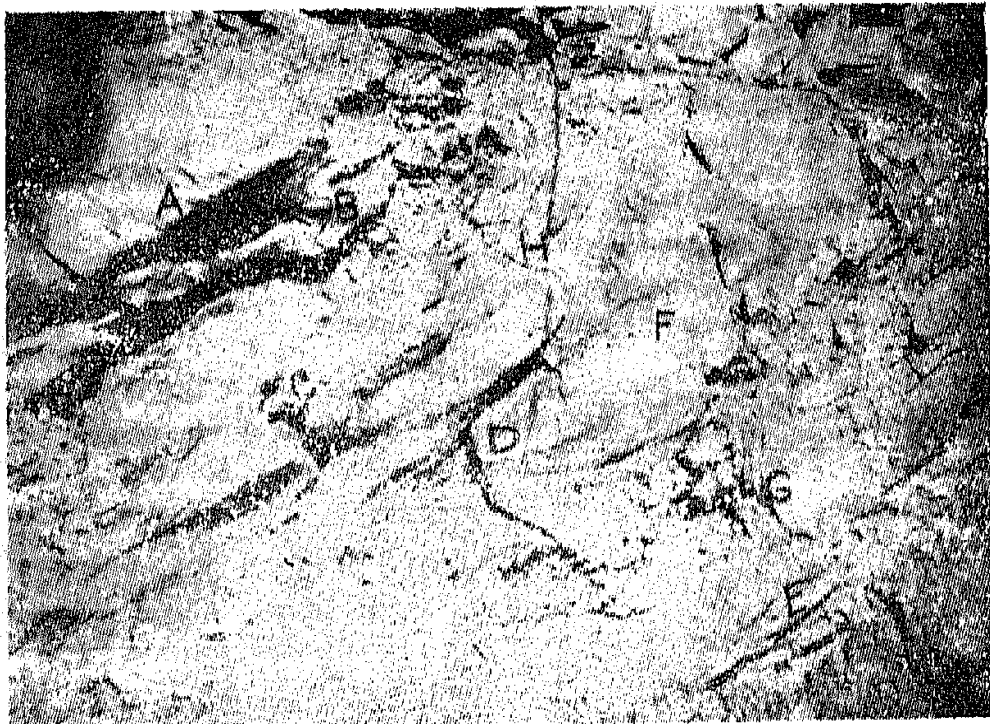
Photo—2. Highly fractured rock zone with excessive fissures and voids
